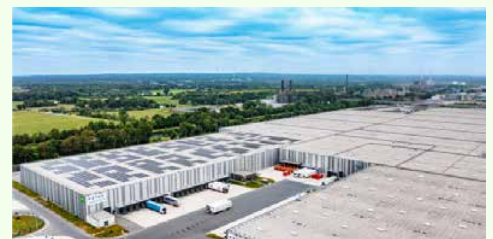
Goodman's largest solar installation globally Marl, Germany
